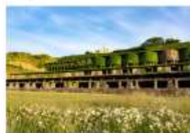
KITAZAWA FLOTATION PLANT
